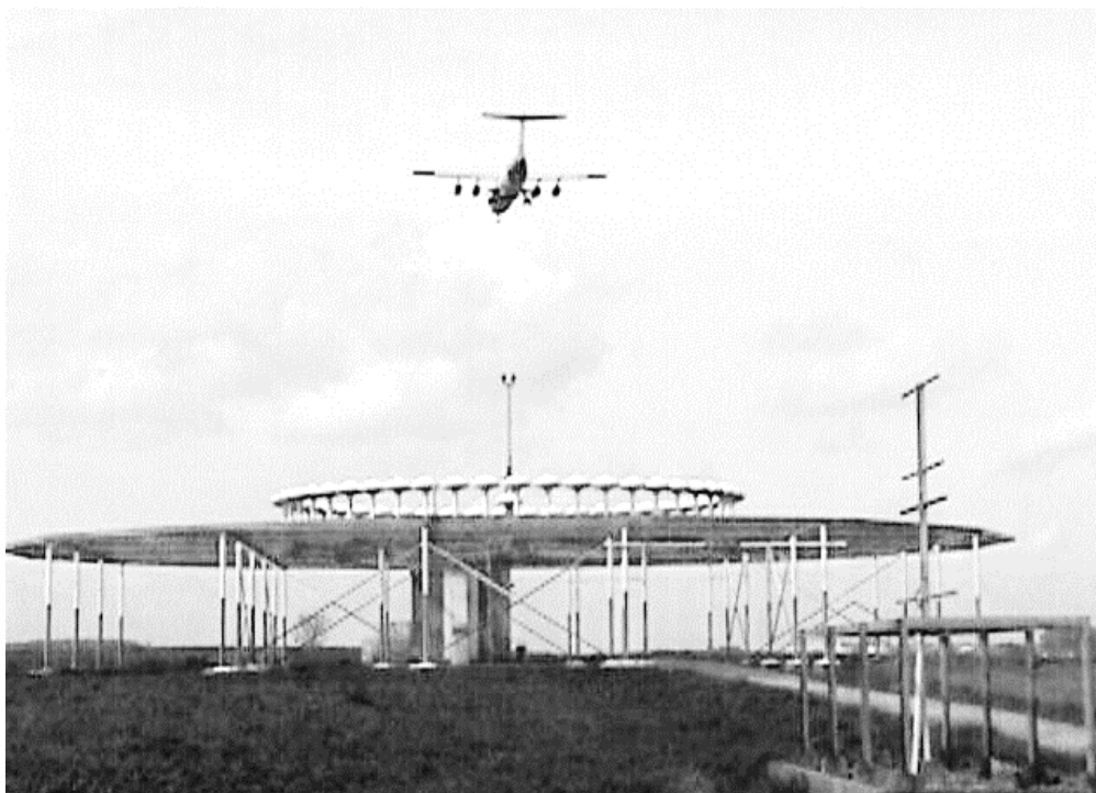
Fig.1 - VOR compatible DME lighthouse
